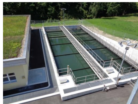
Sedimentationsbecken PAK-Stufe (links Filter)
